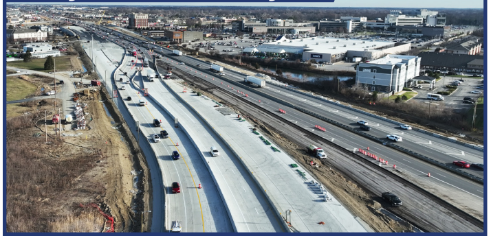
New travel lanes along I-69 South leading into main interchange
